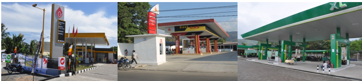
FIGURE 3: 3 NEWLY CONSTRUCTED AUTOMOTIVE FUEL FILLING STATIONS (AFFS) LOCATED IN DILI & MANATUTO
