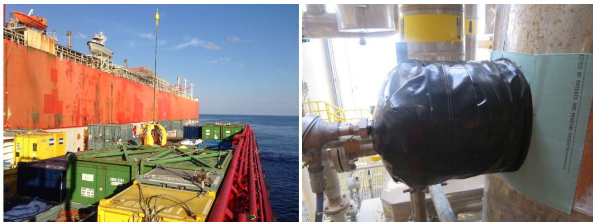
FIGURE 25: MAINTENANCE TEAM TRANSFERRED FROM BU-CPP TO BU-FSO USING FROG OPERATION AND USING STOPAQ PRESERVATION
